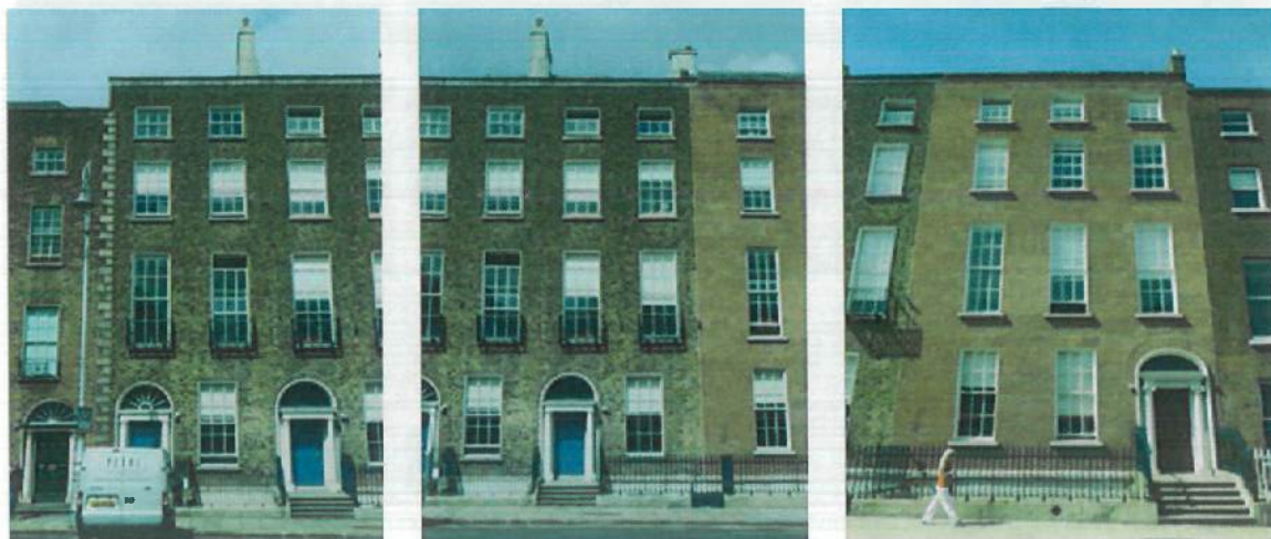
Figure 12. Nos. 91-93 Merrion Square (noted that No. 94 is also owned by the State)
