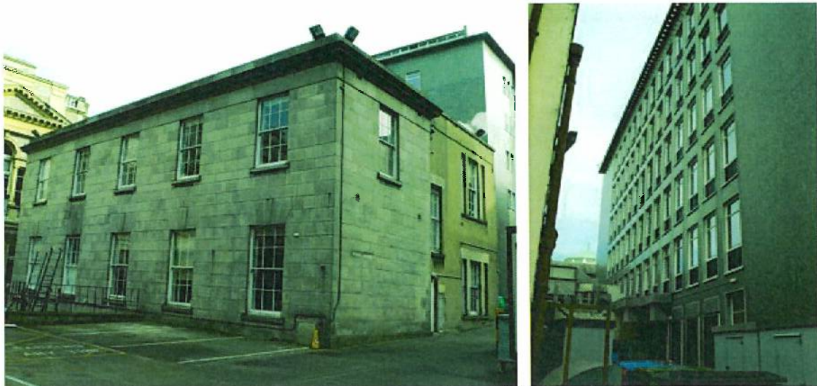
Figure 10. Left Photo: 1930 Block (Image: NIAH); Right Photo: 1966 Block (Image: NIAH)
