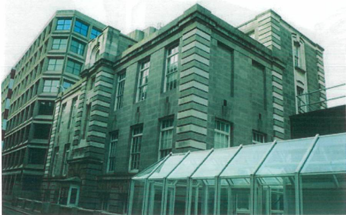
Figure 9. Service Building for Former University Buildings (Image: NIAH)
